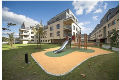
Ostoja-Wilanów (stage 5). Date of delivery: 2010. No. of units: 178 apartments (16,525 sq. m). 13 commercial units (1,212 sq. m).
